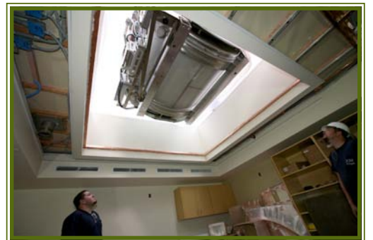
The new 3T MR scanner was lowered into place through the roof of Emory University Hospital.
