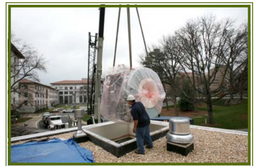
The new 3T MR scanner was lowered into place through the roof of Emory University Hospital.
