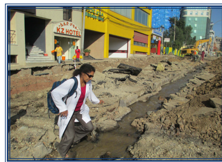
Addis is a growing city with lots of construction. Dr. Sekhar jumps these sewage rivers to get to work.
